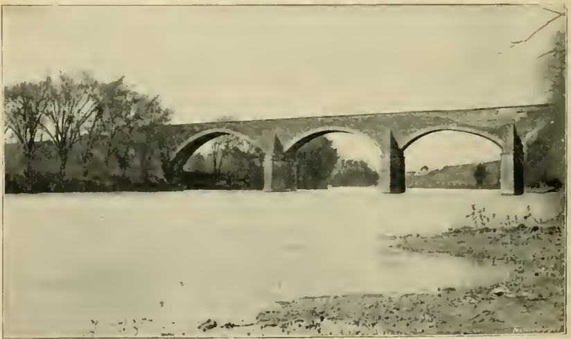
MONOCACY STONE BRIDGE, BALTIMORE PIKE
